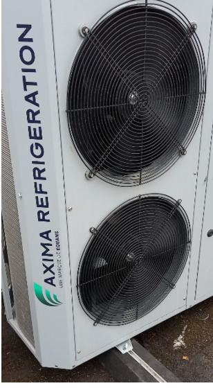
The installation has been split into 2 parallel yet independent systems, in order to obtain R-454C unit charge sizes aligned with EN378 standards. As an added advantage, this configuration offers redundancy and ease of maintenance. The R-454C included the cold storage units, refrigeration production, and all safety elements fully meet current regulations. The refrigerant itself was supplied by Gazechim Froid.
