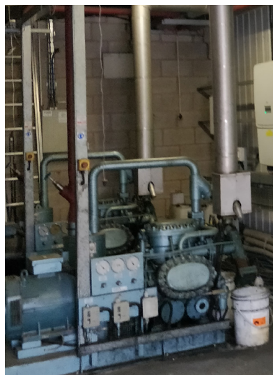
Legacy Grass RC69 Compressor and Evaporator arrangement over loading bays.
