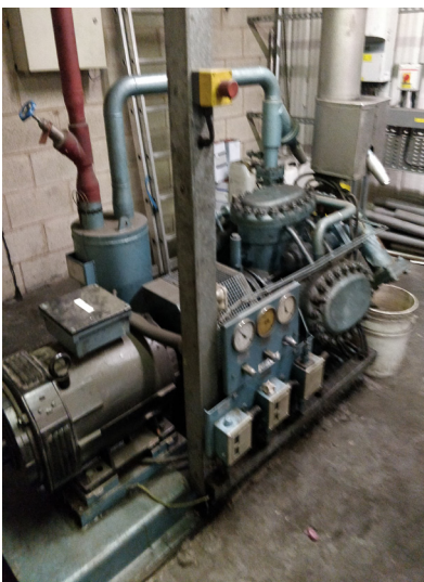
Legacy Grass RC69 Compressor and Evaporator arrangement over loading bays.
